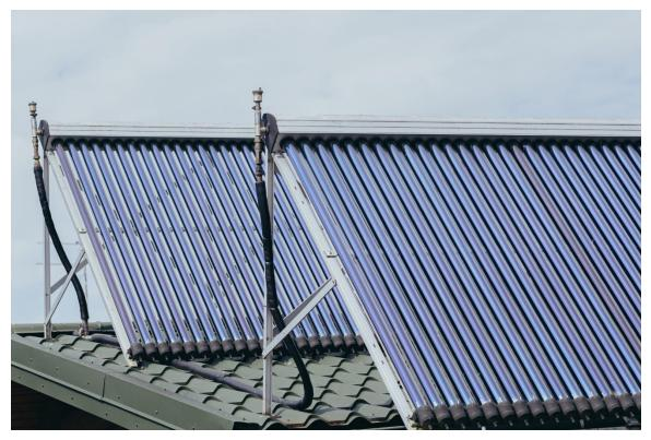
Solar water heating systems, or solar thermal systems, use energy from the sun to warm water for storage in a hot water cylinder or thermal store. Because the amount of available solar energy varies throughout the year, a solar water heating system won't provide 100% of the hot water required throughout the year. A separate system, usually your existing boiler or other water heating system, is used to make up the difference.
